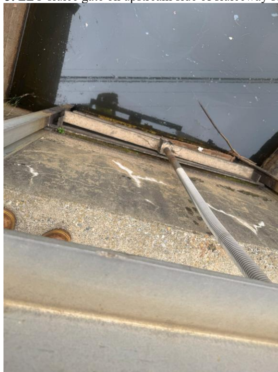
Photo 3. LLO sluice gate on upstream side of sluiceway structure
